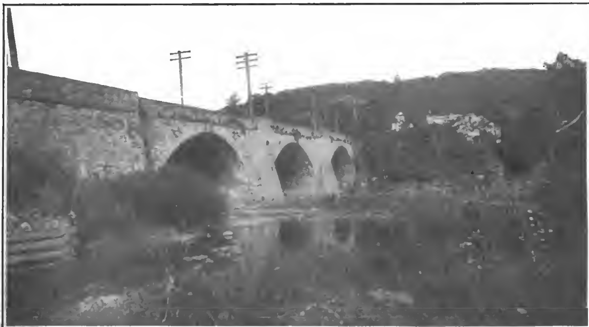
STONE ARCH BRIDGE ACROSS THE YOUGHIOGHENY RIVER AT SOMERFIELD, PA., BUILT IN 1818.
